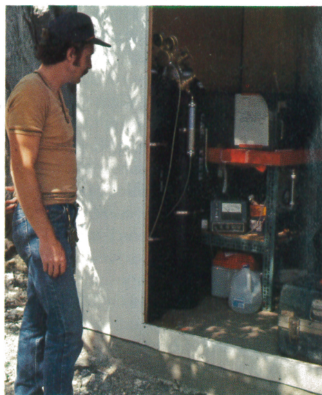
(above, left) The Pacoima Dam is located (facing page) in a gap in the San Gabriel Mountains near San Fernando, California. (center) Just around the bend from the dam, the Gulf van is parked near the shed that houses the Caltech-Gulf monitoring instruments. (right) Gulf Technician D. J. Masdea inspects the gas chromatograph. The high degree of automation employed makes such visits infrequent.
